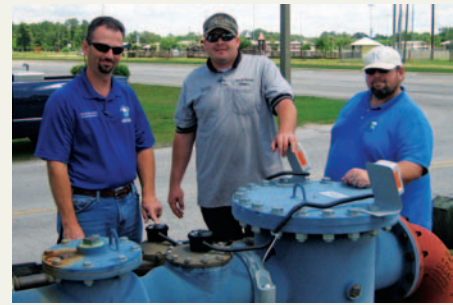
Inspecting installation of 10" HP PROTECTUS III (L-R): Rhett McCamey (Superintendent), Brandon Richardson (Foreman), Shawn Ladd (Supervisor).
