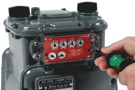
Figure 5 Index Removal
