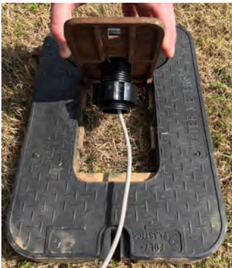
Figure 30 – Securing the Locking Nut
