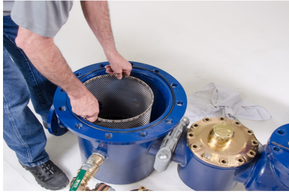
Figure 34 – Replacing the Basket
