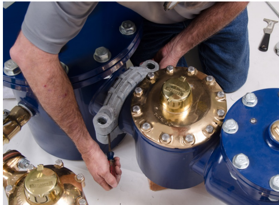
Figure 56 – Loosening the Coupling
