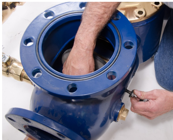
Figure 50 – Inserting the New Bolts
