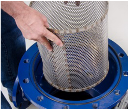
Figure 21 HP FS Strainer Basket
