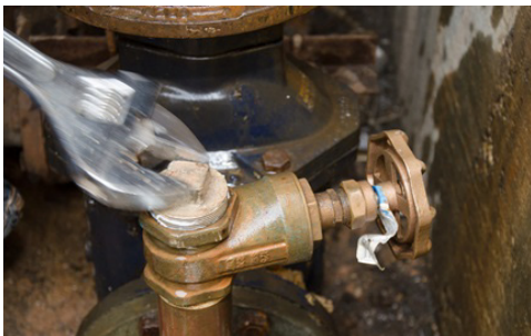
Figure 4 Remove Test Plug
