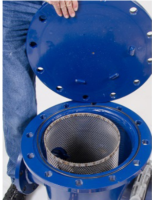
Figure 20 HP FS Strainer Cover
