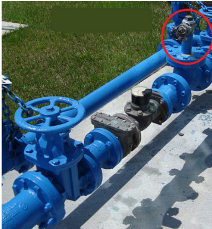
Figure 2 HP Turbine with Test Tee Installed
