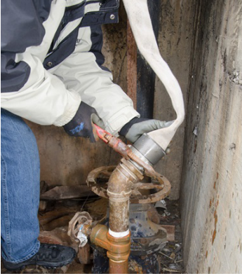
Figure 5 Connect Fire Hose to Meter Under Test
