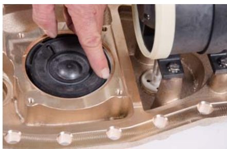
Figure 24 Placing the T-10 Chamber
