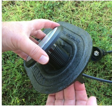
Figure 22 – Inserting Antenna into Pit Lid
