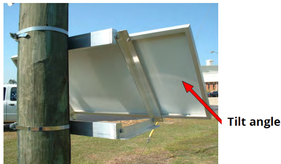
Figure 55 – Mounted Solar Panel
