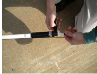
Figure 77 – Weatherizing RF Antenna
