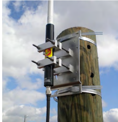
Figure 48 – Coaxial Cable Attached
