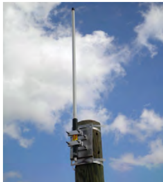
Figure 47 – RF Antenna Bracket
