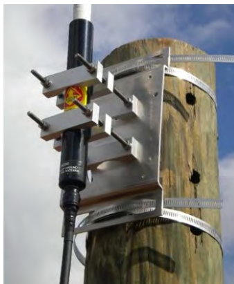
Figure 49 – Weatherized Connection
