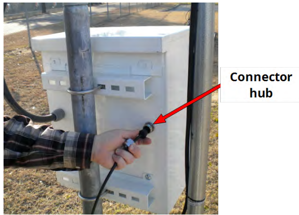
Figure 37 – Feeding Conductor Wire
