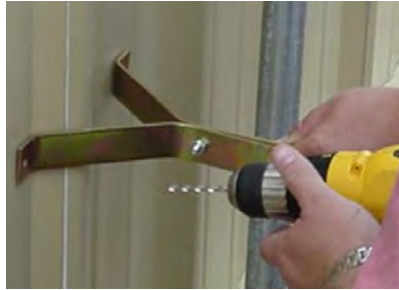
Figure 74 – Lining up Second Pole Bracket
