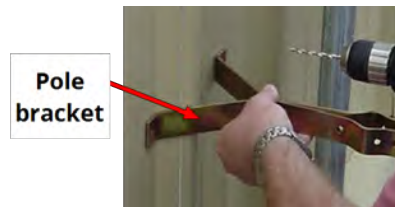
Figure 73 – Securing Pole Bracket
