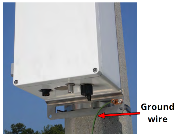
Figure 57 – Attach Ground Wire
