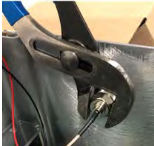
Figure 107 – Remove Existing External Cellular Antenna
