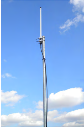
Figure 79 – Securing the Coaxial Cable
