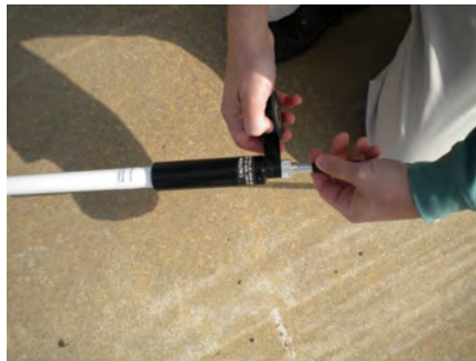
Figure 26 – Weatherizing the RF Antenna
