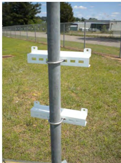
Figure 28 – Installing Pole Brackets
