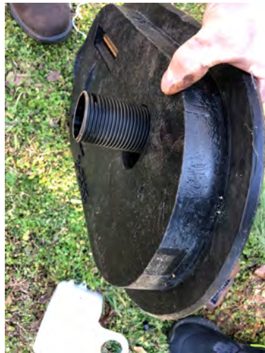
Figure 43 – Insert the Flange Tube
