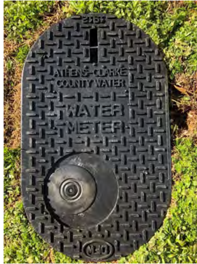
Figure 51 – Replace the Meter Lid
