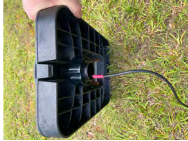
Figure 54 – Antenna Installation Complete
