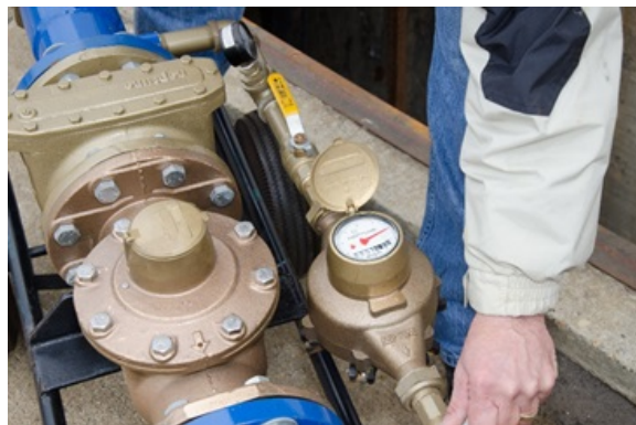
Figure 7 – Release Trapped Air – Low Side
