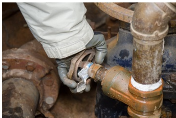
Figure 5 – Gate Valve
