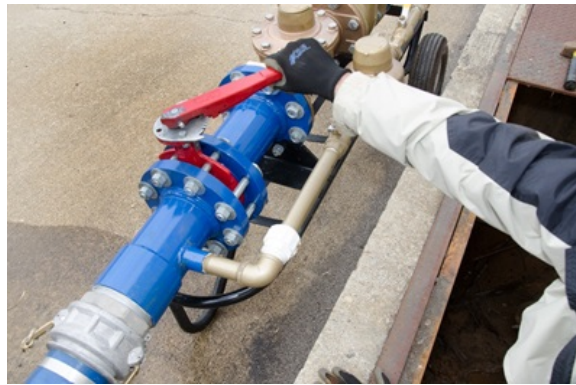
Figure 6 – Release Trapped Air– High Side
