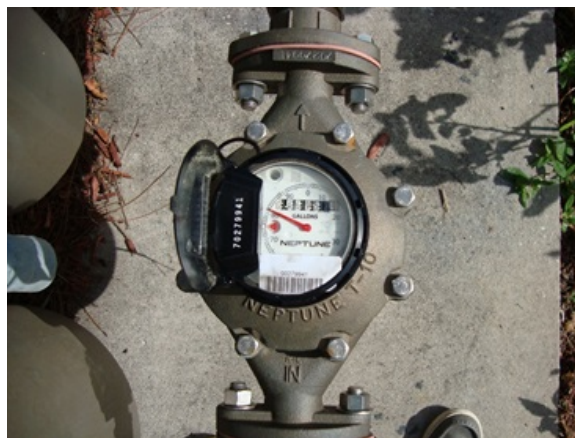
Figure 9 – Register – Low Side
